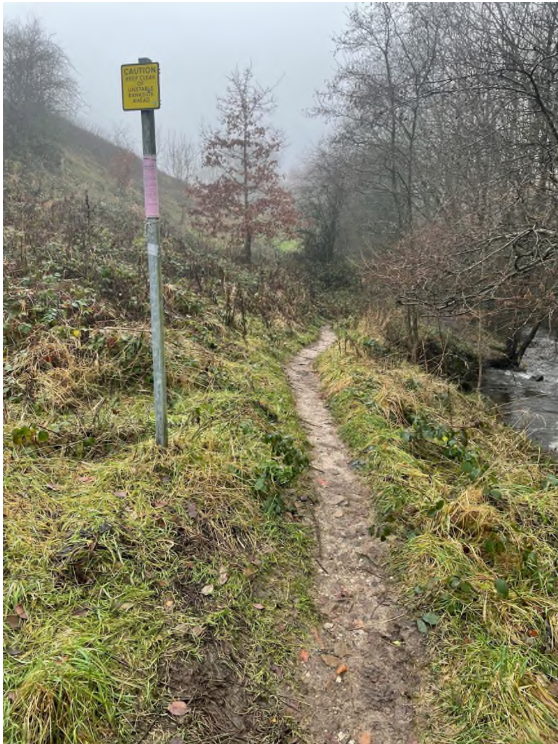
Photograph 21: Shows the track leading to the junction with Footpath 25 and sign stating “Caution Keep Clear of unstable bank side ahead”
